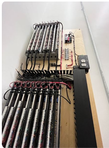
Pipe drivers, which serve as the electrical connections between the pipes and the console.
