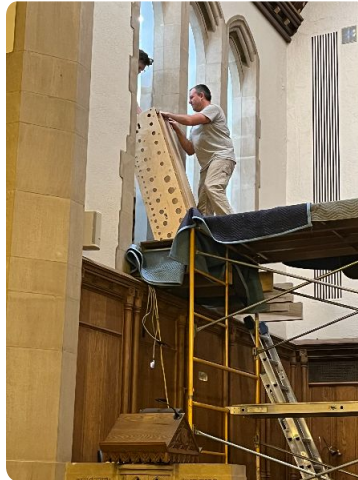
A windchest going into the Choir Chamber (left side of Chancel).
