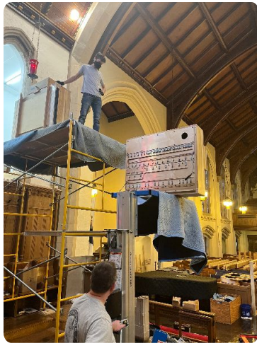
Scaffolding was erected and a lift used to bring the windchests and other parts to the chamber openings.
