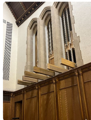
These wood beams will provide structural support for the wood casework and pipes that will be visible in the Chancel.
