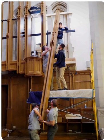
More casework beam placement. (Photo credit: John Mitchell)
