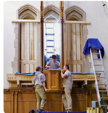
The center "tower" of the casework is raised into place. (Photo credit: John Mitchell)
