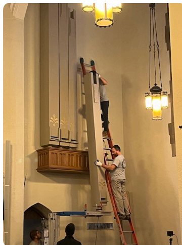
Each Open Wood pipe was hoisted up with the help of a power lift, and then manually put into place.
