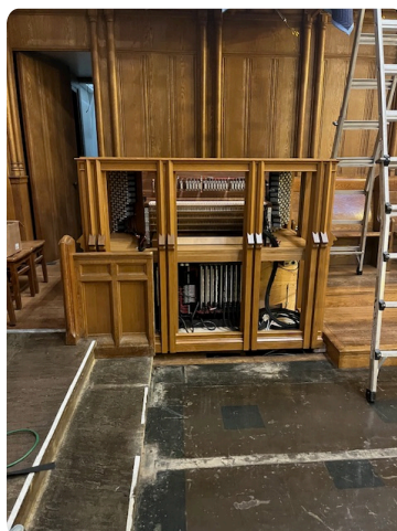
Console installation in the Chancel. Many miles of wiring
