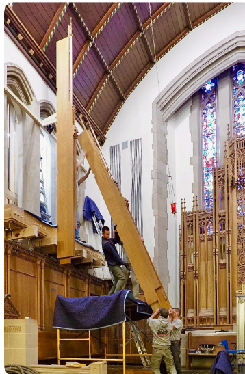
The Zimmer team raises the large oak beams for the casework. (Photo credit: John Mitchell)
