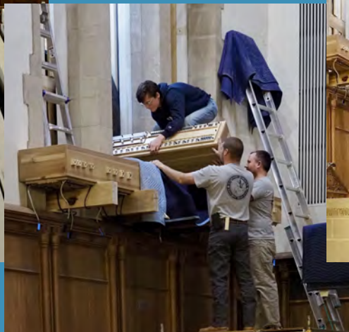
A windchest going into the chamber through the arch in the Chancel wall. (credit: John Mitchell)
