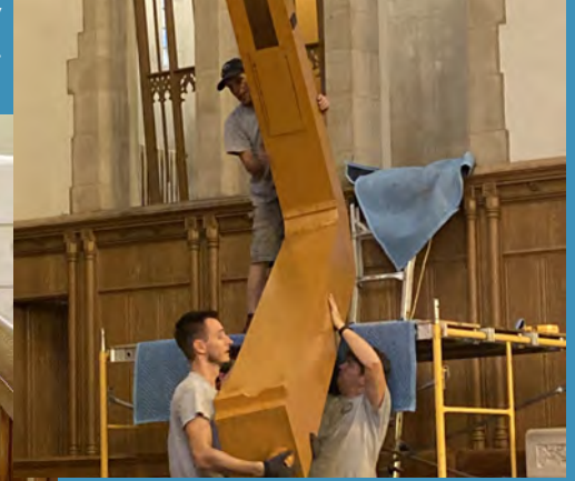
One of the largest Open Wood pipes is removed from the chamber. Mitered to fit in the chamber, the Open Woods were straightened and now reside on the transept walls on each side of the Chancel. (credit: Joyce Summers)
