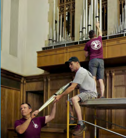
The Zimmer Organ team removes pipes from the exposed wind chests in the Chancel in August 2022. (credit: John Mitchell)
